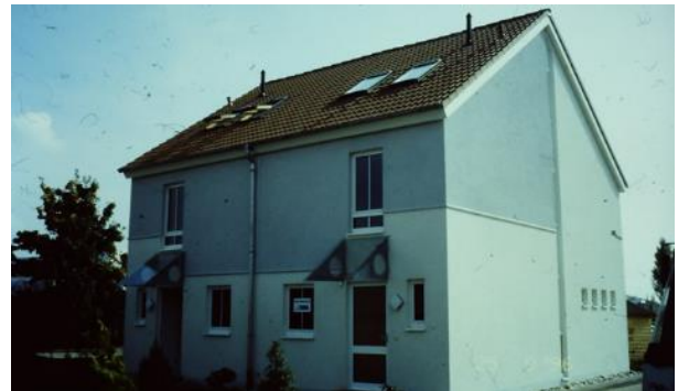
Figure 9. The built "x8 Haus" applying the ROD concept (Photo: T. Bock)
