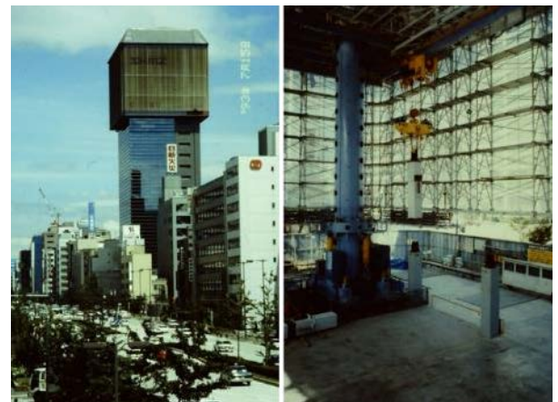
Figure 3. The pioneering automated construction site “SMART” developed by Shimizu Corporation (photo: T. Bock)
