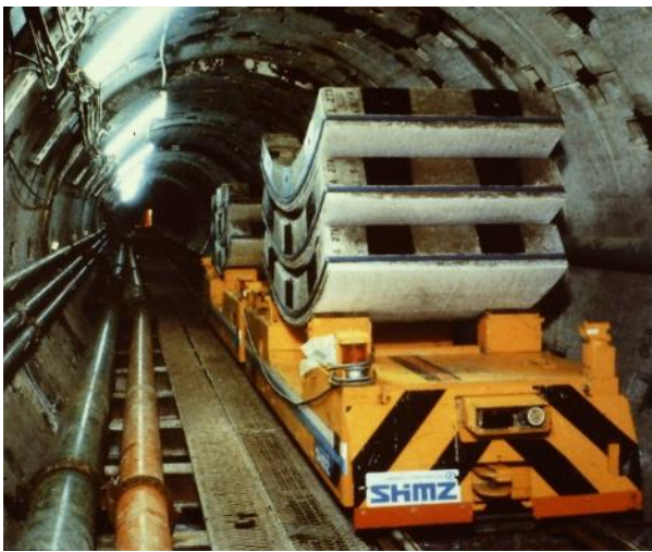
Figure 4. Teleoperated construction robot for concrete tunnel construction (photo: T. Bock)
