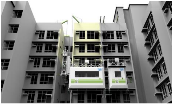
Figure 10. The multifunctional façade-processing robot showcasing the painting function on the façade of public housing buildings in Hong Kong (image: R. Hu)
