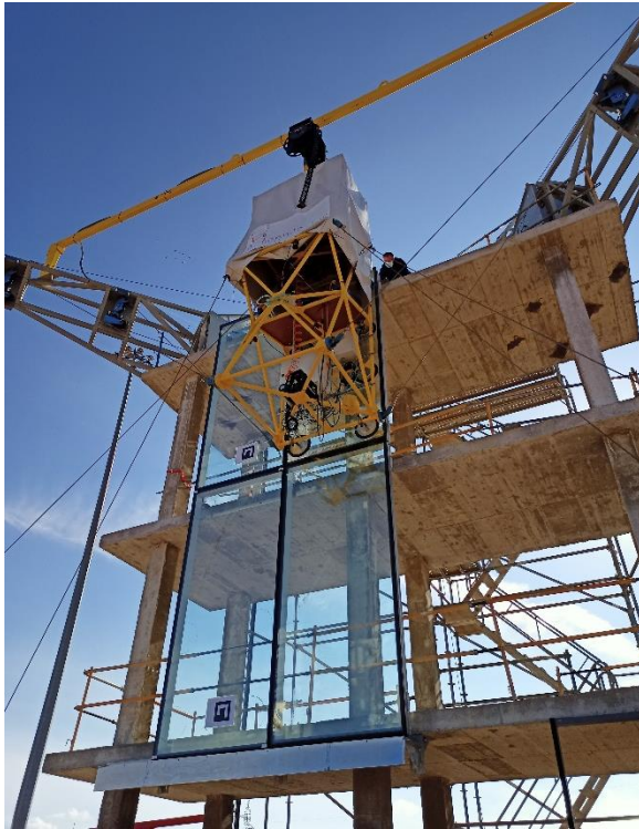
Figure 12. The HEPHAESTUS cable-driven façade installation robot on a testing site (photo: K. Iturralde)
